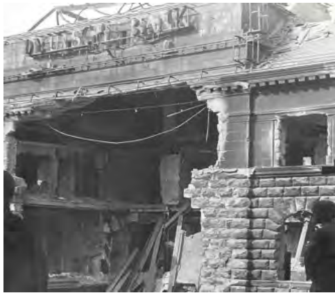
Damaged Deutsche Bank's head office in Berlin
