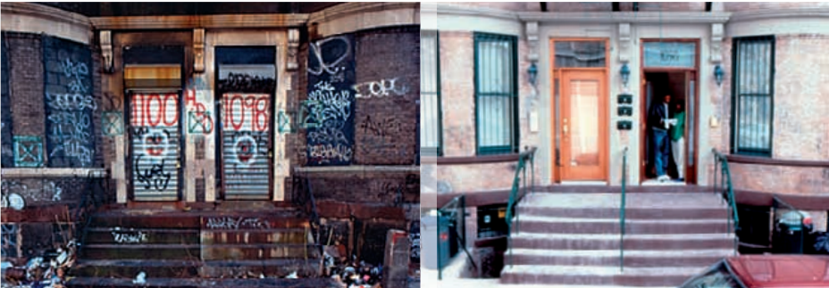
From ruins to high-quality living quarters: buildings on Jackson Avenue, South Bronx
